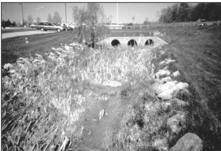
Figure 4.6.1-3. Moderate Channel Alteration Problem
