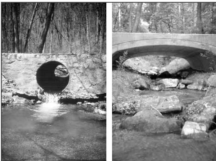
Figure 4.6.5-4. Perched culvert before and after restoration project.
