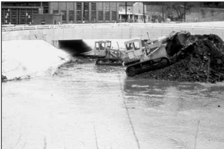
Figure 4.6.7-1. An instream construction site.
