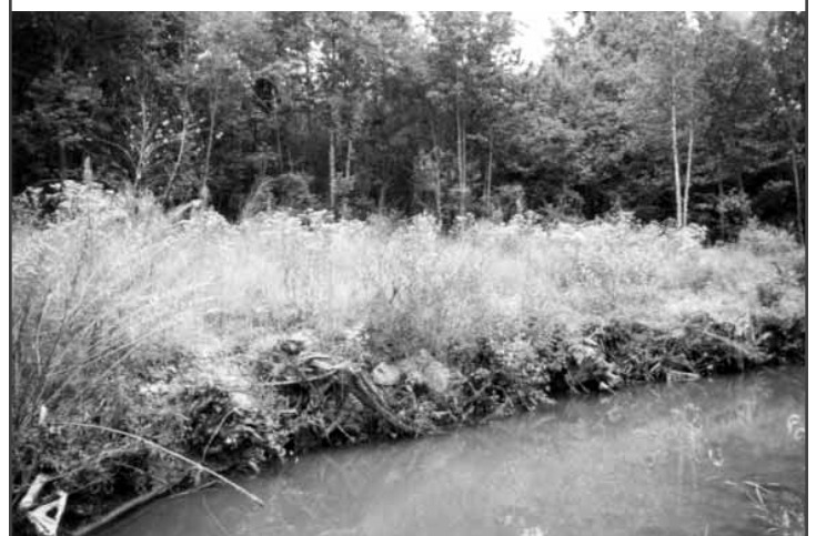
Figure 4.6.3-3. Exposed pipe before and after stream restoration project.
