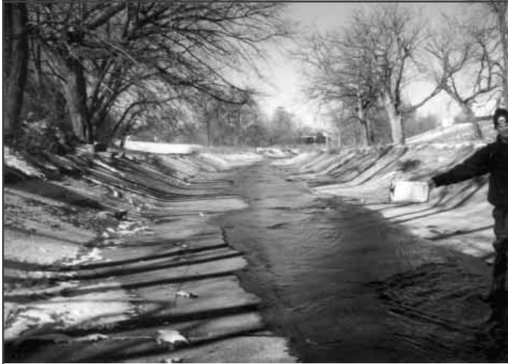
Figure 4.6.1-2. Severe Channel Alteration
