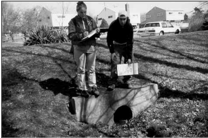
Figure 4.6.4-3. Minor pipe outfall site.
